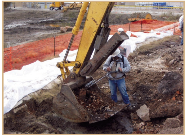
Real time monitoring of contaminated soil.
