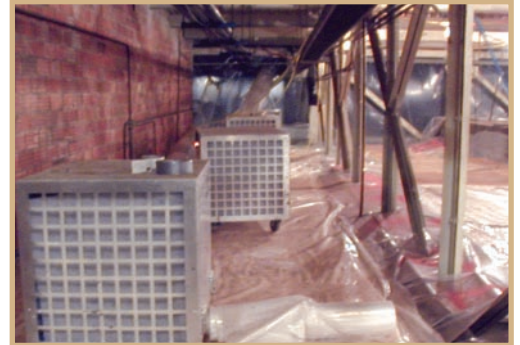
Negative air units used during PCB contaminated lead paint removal.
