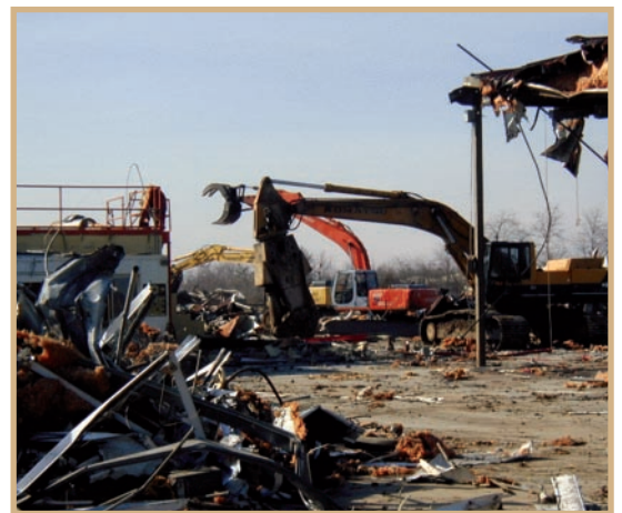
Demolition of former manufacturing facility.
