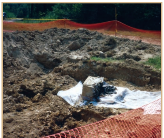
Removal and disposal of batteries at former defense firing range.
