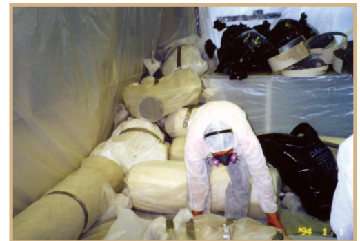
Asbestos abatement at office building.
