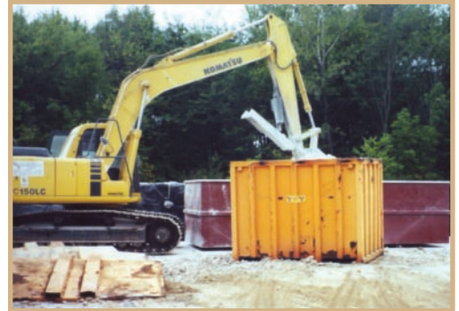
Stabilization of high moisture content waste prior to disposal shipment.
