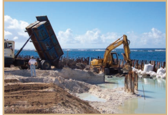
Excavation of PCB-impacted soil on Pacific Ocean atoll.
