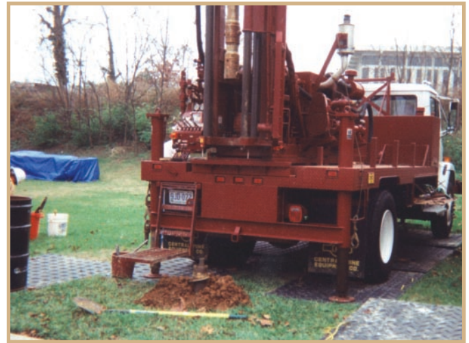
Chase drilling crews provide experienced personnel to support site investigation activities.
