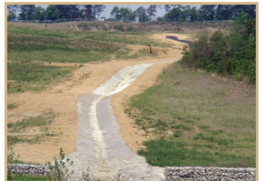
Repairs to CERCLA cap.
