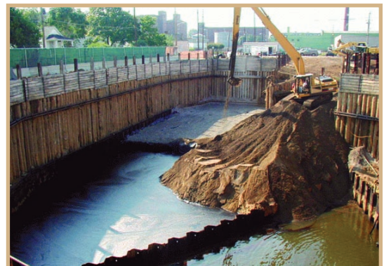
Removal of petroleum-contaminated soil below groundwater table.
