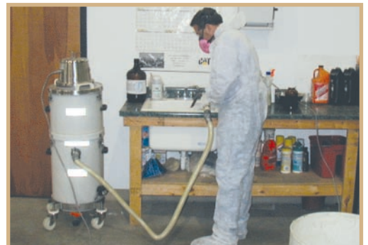
Remediation of laboratory drain contaminated with mercury.
